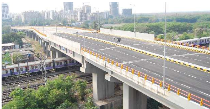
New Dahisar Bridge
